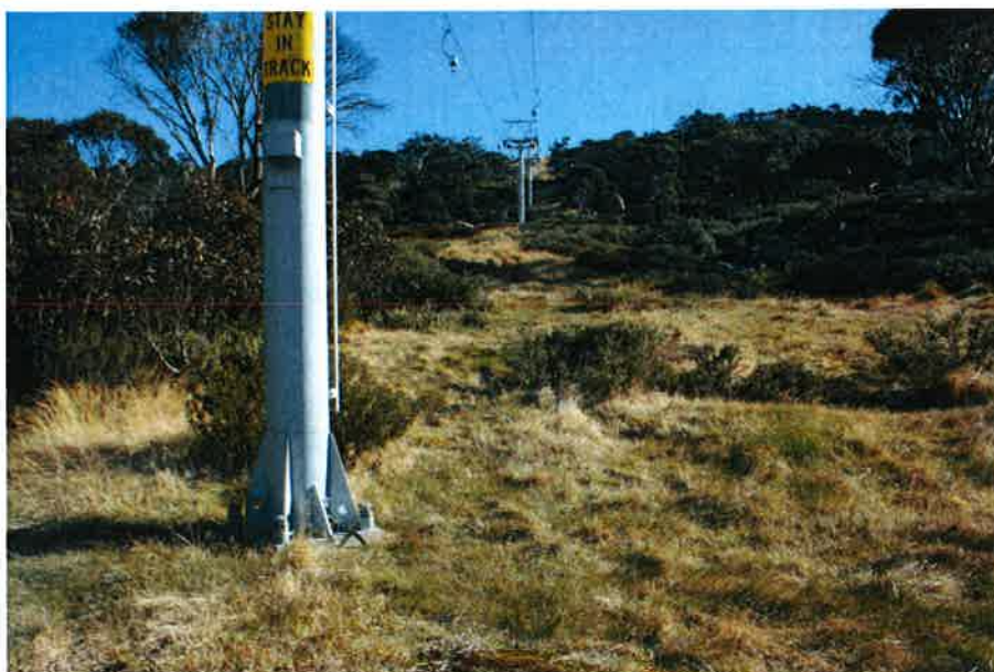
Photograph 3: View upslope with Tower 1 in the foreground.
